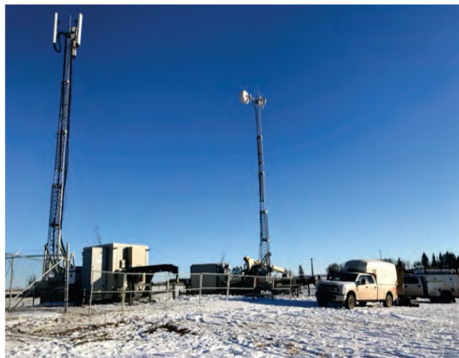
WesTower Communications deploys cell site on wheels in Eden Valley, AB
